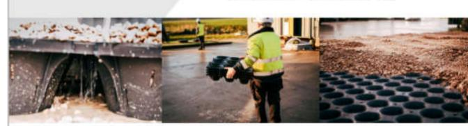
Formavoid is a plastic void former that encourages fill material into an extremely strong series of columns and catenary arches. Formavoid can be filled with various materials ranging in particle sizes from 1mm - 40mm. Different fills can be used for various characteristics & applications. For example, 30% void type 3 aggregate is optimal when utilising formavoid in a subbase attenuation applications; or soil can be used as fill material for green infrastructure applications.
